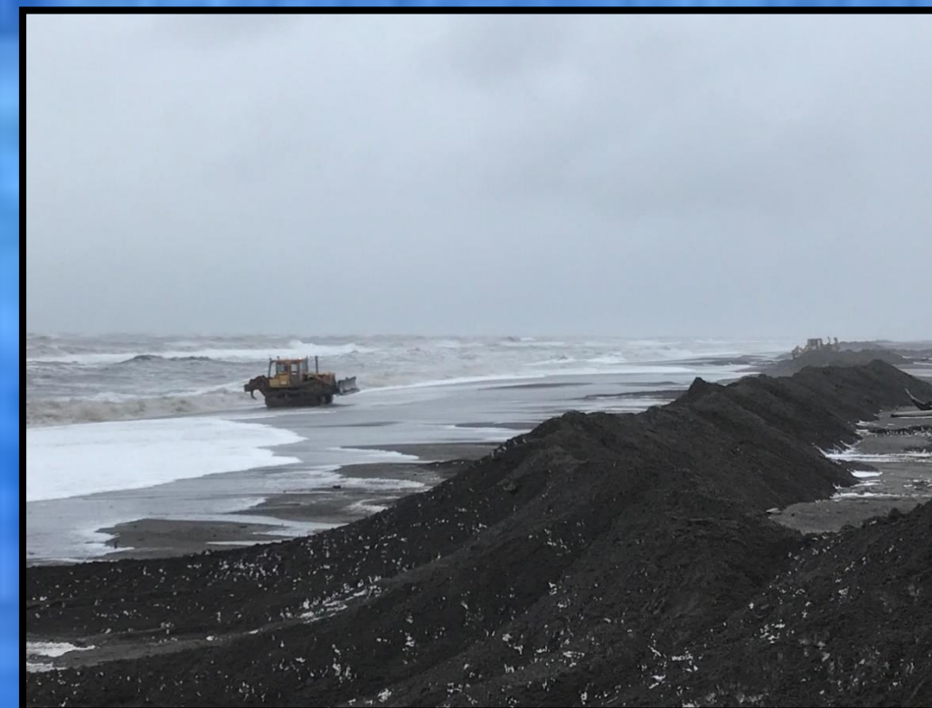
Emergency Sea Wall, Utqiagivk, Pic: North Slope Borough
